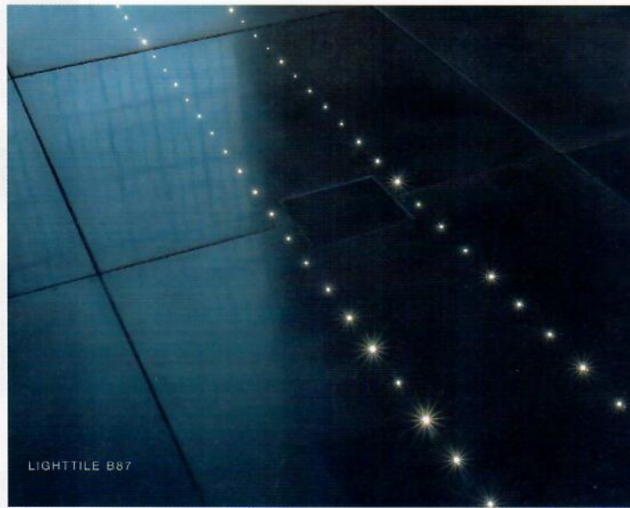
Siut GmbH has developed concrete floor tiles with integrated optical fibers that are used as an esthetic enhancement on the one hand and as a medium of communication on the other
