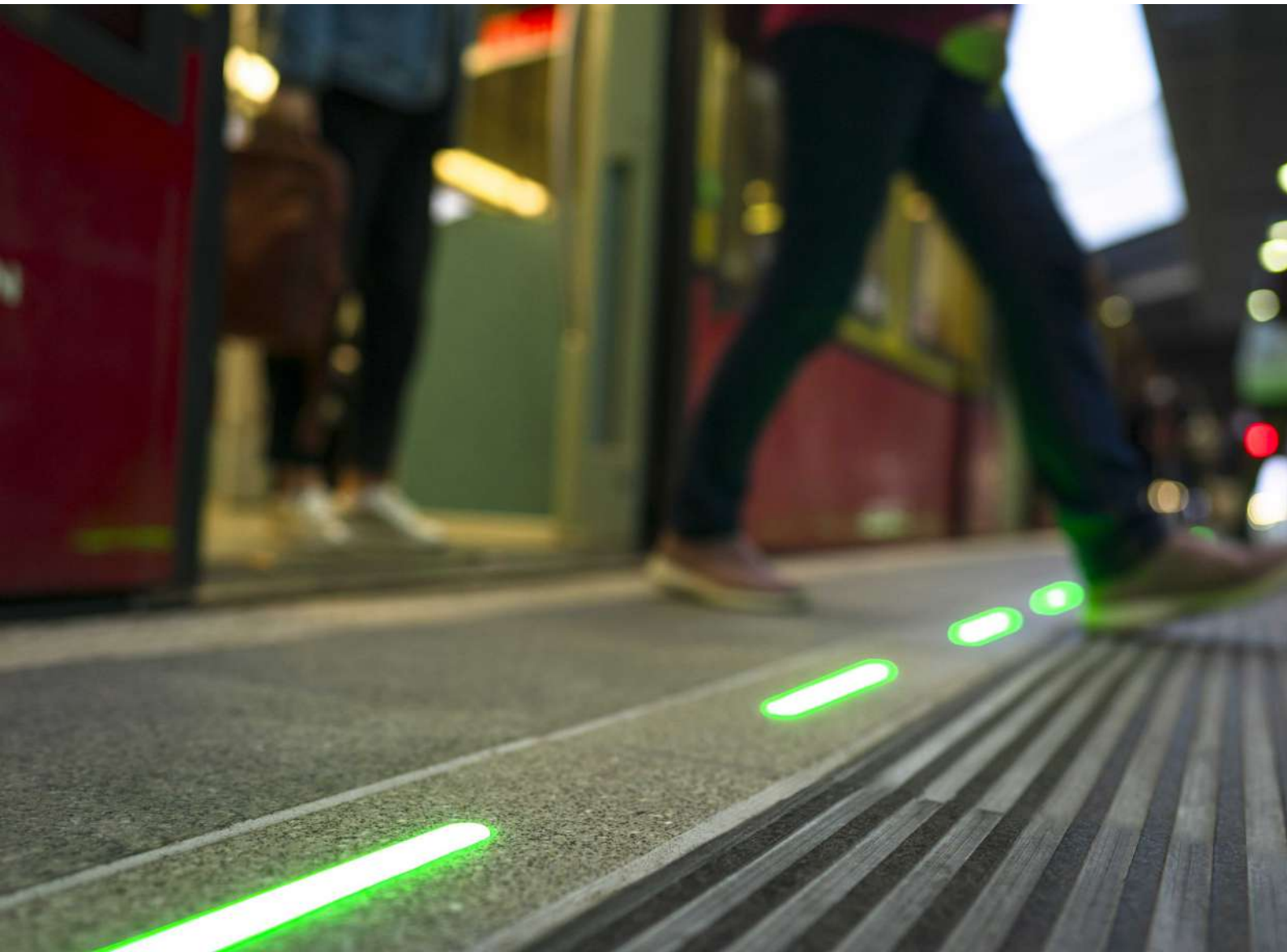
Illuminated Platform Edge
