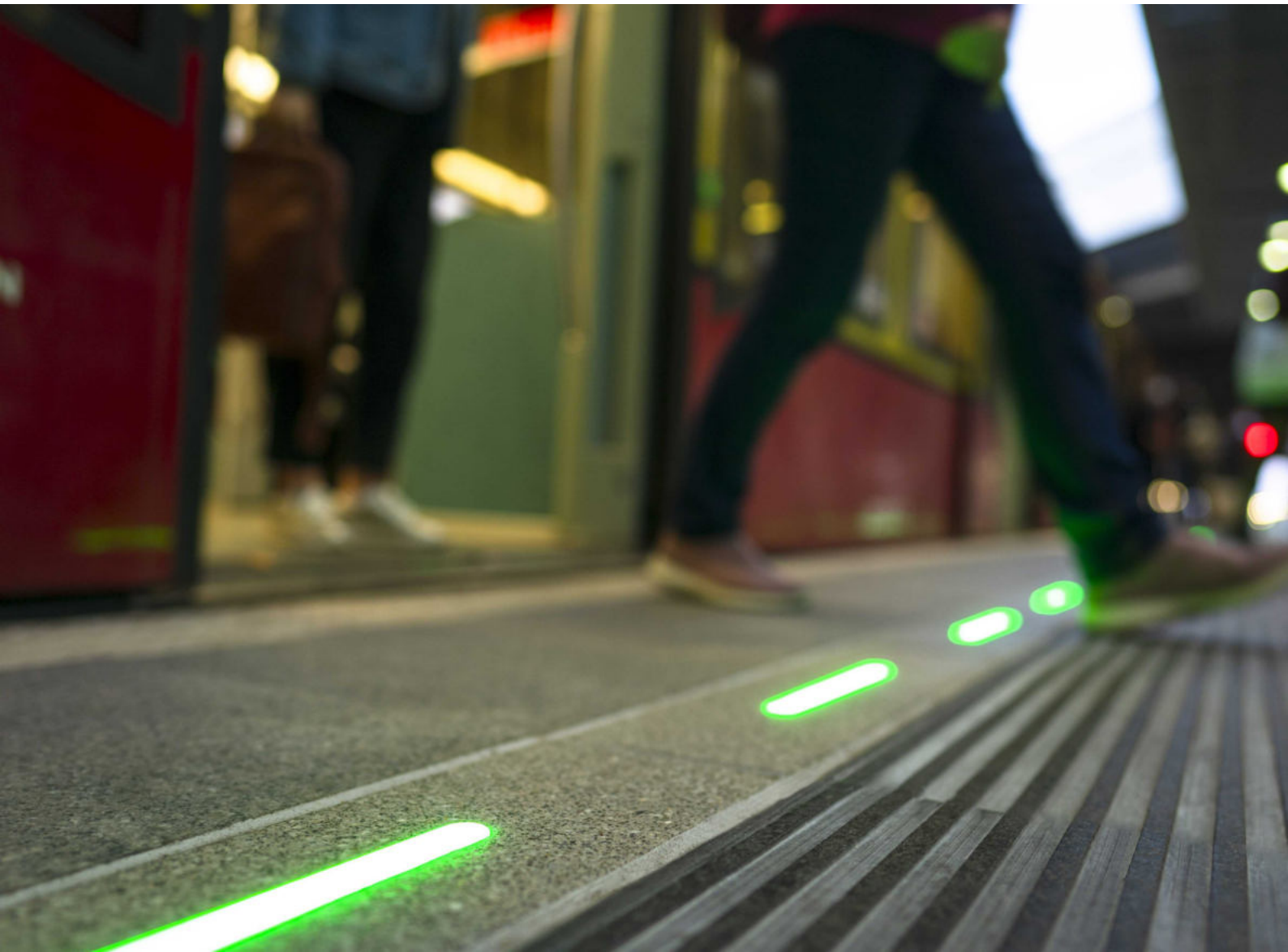
Illuminated Platform Edge
